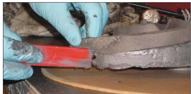
Repairing a pump impeller with Loctite® Fixmaster® Wear Resistant Putty
