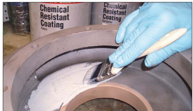
Coating a pump volute with Loctite® Nordbak® Chemical Resistant Coating
