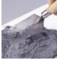
Epoxy is turned out onto a disposable surface to ensure proper mixing
